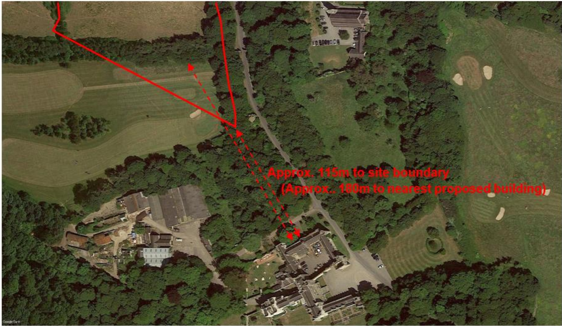
Plate 3 Howth Castle & Associated Building relative to proposed development site
